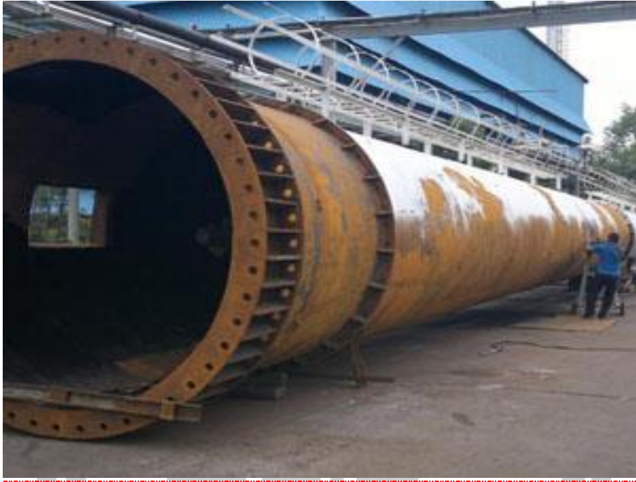
CHIMNEY FABRICATION WORK
