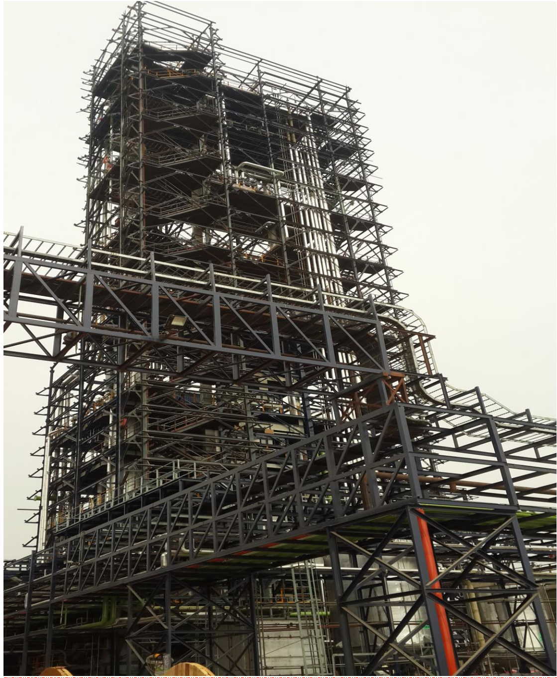
PIPING WORK UPTO 65Mtr. Level.
